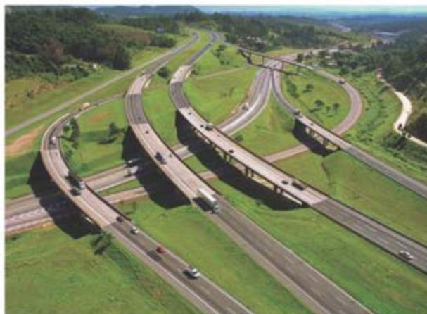
State highways under concession: to build an access, authorization from Artesp is required.
